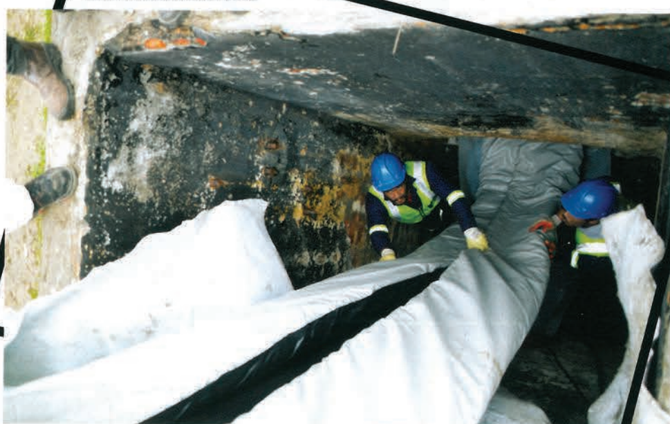
Installation of liner in Black Mac Sewer
