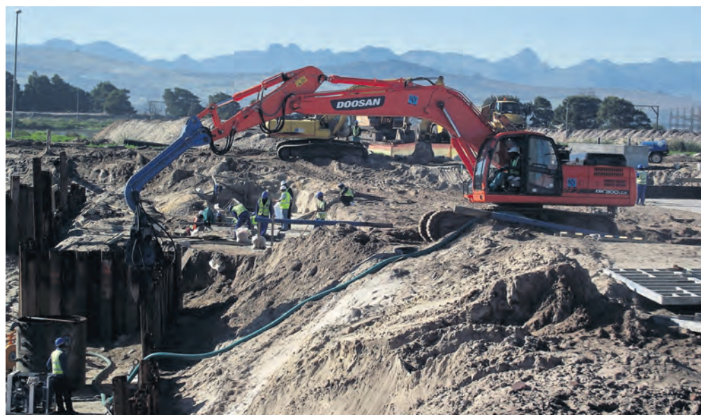
Temporary shoring being installed at the Bellville Waste Water Treatment Works in 2011 to retain a large sewer pipeline for a deep excavation.
