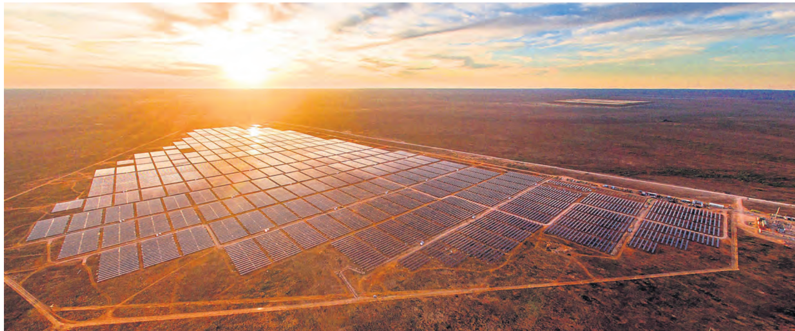
The Mulilo Sunpower 75MW Solar PV project at Copperton in the central Karoo.
