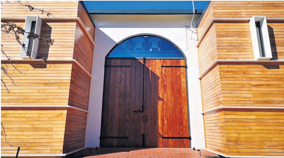
CSV completed the Taabosch cellar (formerly Cordoba), along with the farmhouse, roads, and related civil infrastructure.
