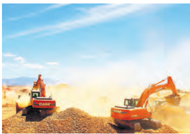
Ground being reworked during one of CSV's projects.
