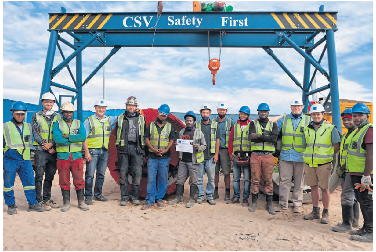
CSV is driven to secure the safety of their staff. Some of the members at the microtunneling machine site in Mitchells Plain.
