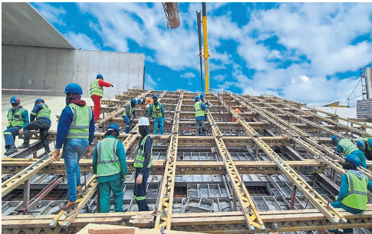
Throughout this project CSV employed various foreman and workers on site.
