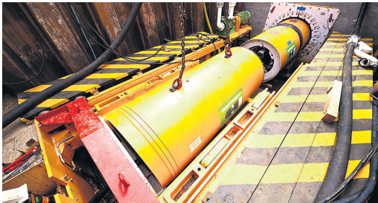
The microtunneling machine installed in Mitchells Plain in October 2020.
