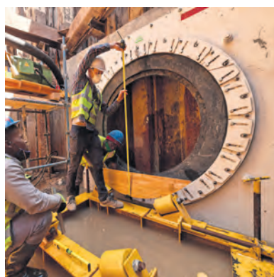
Microtunneling machine site prep being done in Mitchells Plain.
