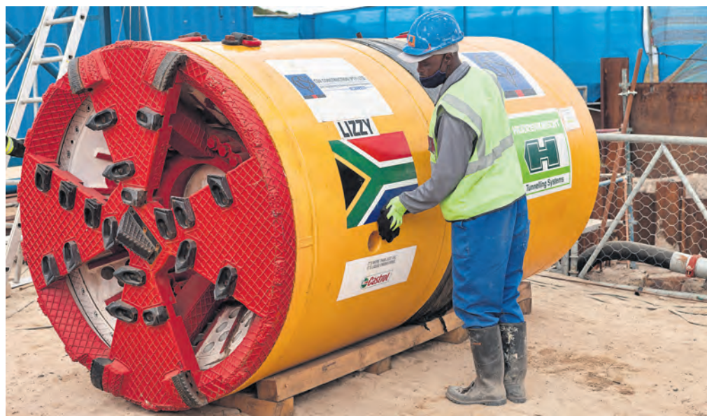
Microtunnel machine prep before installation.
